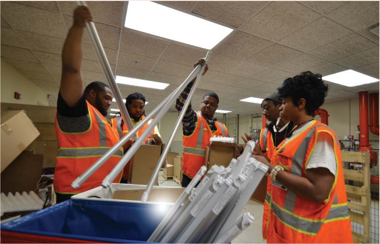
An Evergreen Energy Solutions team installs LEDs in a Cleveland Clinic parking garage, saving money and reducing energy consumption. (Photo: Lisa Chamberlain)
